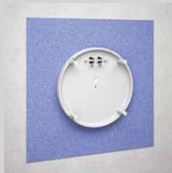
2. Fix sealing fabric on ready plastered and pre-treated wall.
