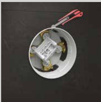
4. Trim the protruding part of the box, turn off the water and disassemble the flushing device.
